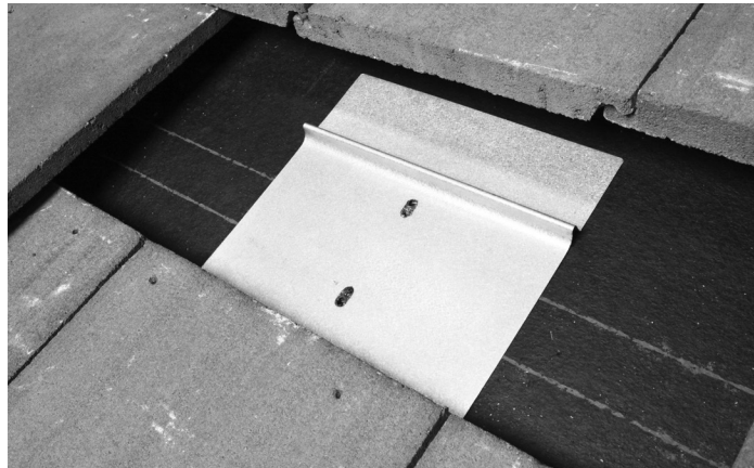
Base Flashing before lag screws installed or sealant applied
