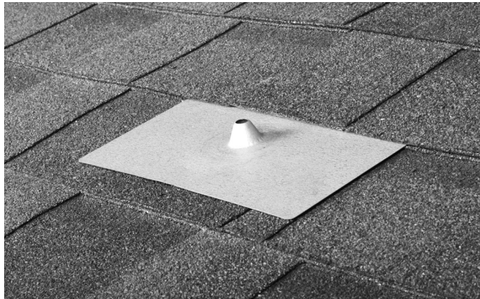
Flashing installed
