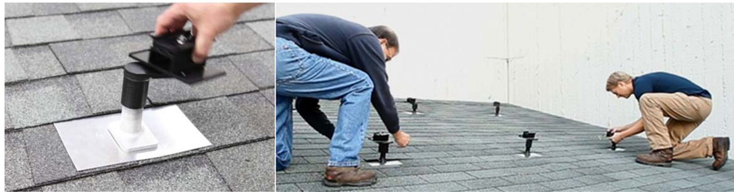
Spin mounting assembly onto base. 8 – turns for single 12 – turns for double
