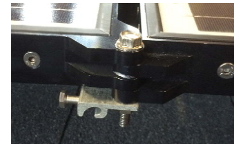
Middle location– 5/16" stainless steel lag bolt and nut.
