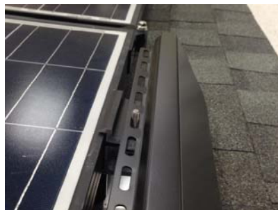
Clamp skirt to front clamp
