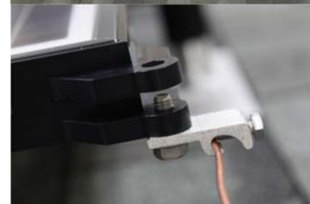
Install lay in ground lug with 5/16" stainless steel lag bolt
