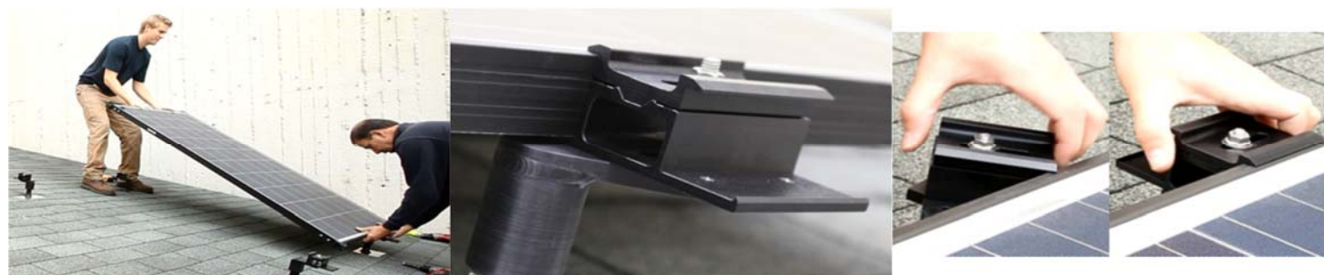
Lay module into first clamp.
