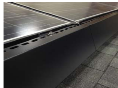
Finished Front Skirt
