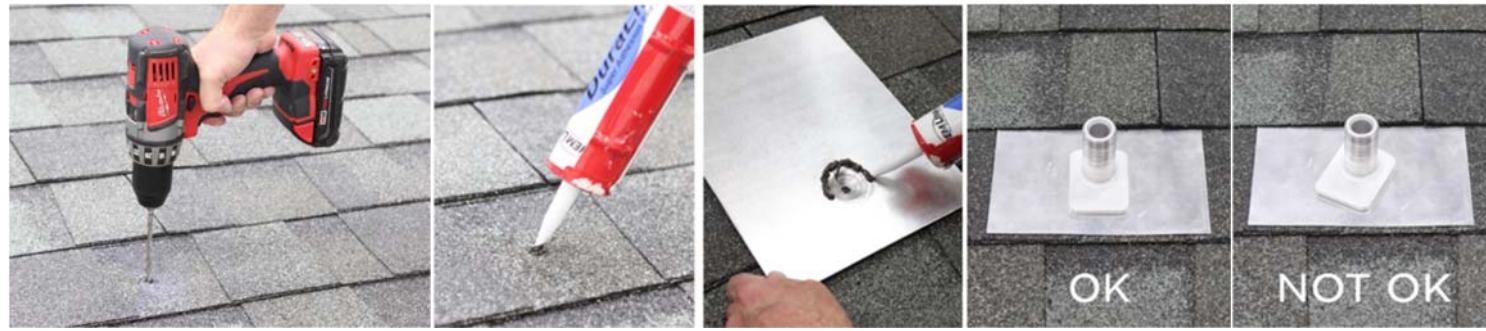
Drill pilot hole with 7/32" drill bit
