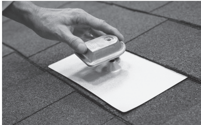
Installing Support Block on LightSpeed Flashing
