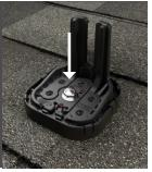
If screw hits rafter, drive second screw in hole above. Ensure screws are embedded at least 2.5" into rafter. Installation complete.
